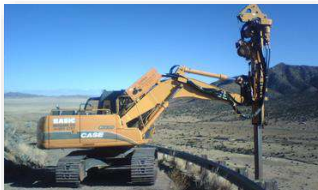
Foundation Drilling
