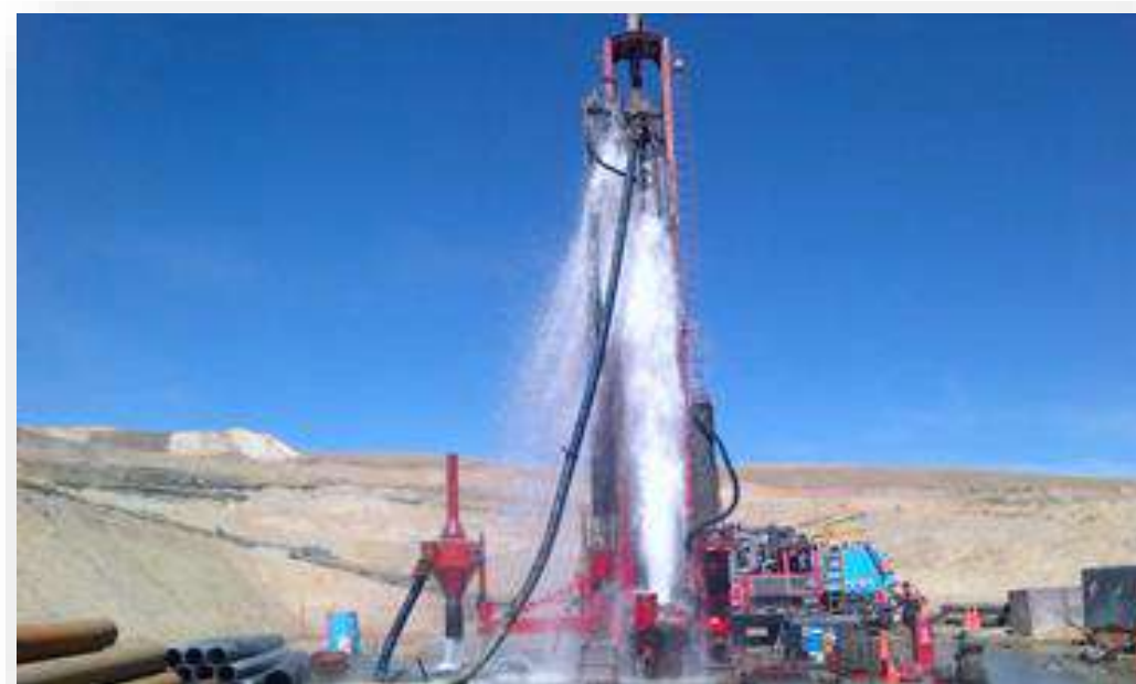
Water Well Drilling
